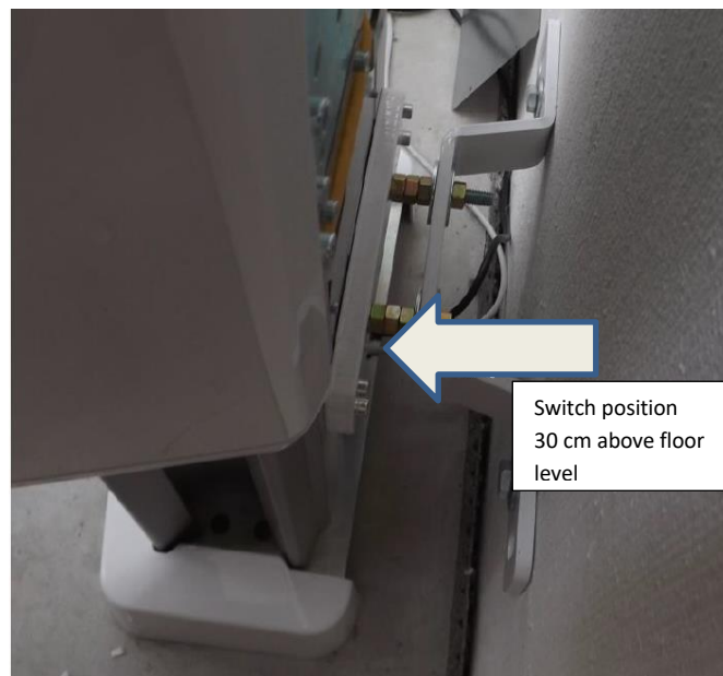
Figure 5 Place of wiring connections
